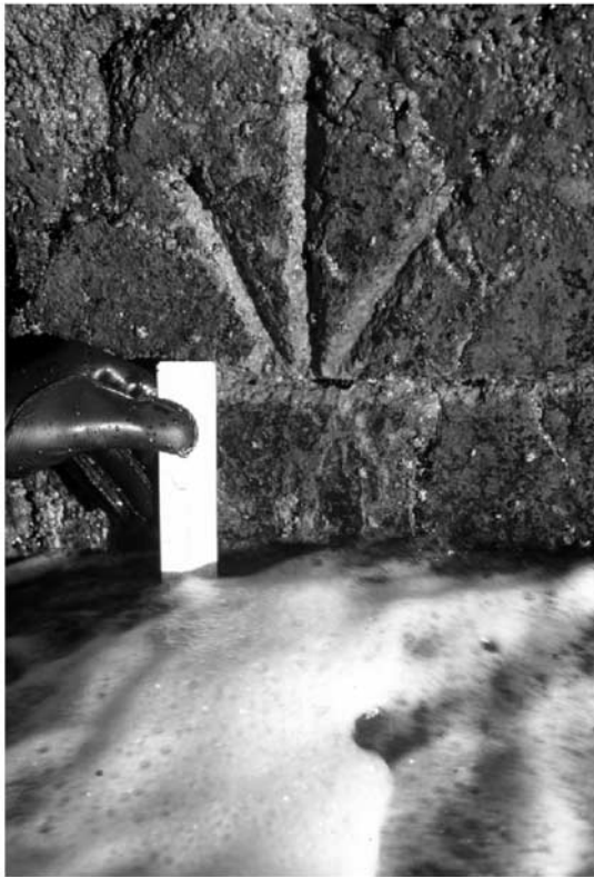
Figure 1. The benchmark on the Isle of the Dead, Port Arthur. The horizontal line is about 0.4 m long.
